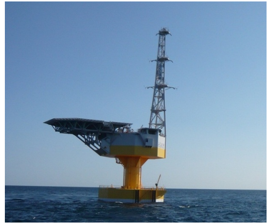
66kV Floating Substation “Fukushima Kizuna” (Floater: Advanced Spar)
